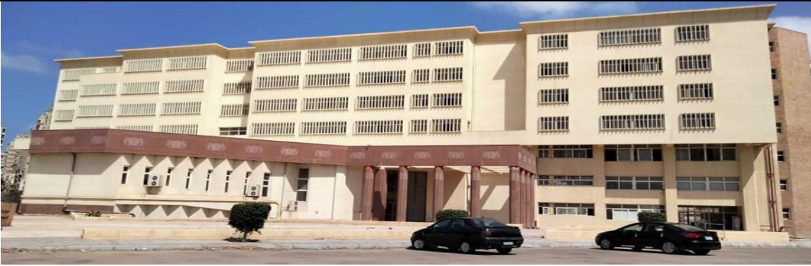
Green building implementation through the use of sun breakers in the SSP building at the Faculty of Engineering
