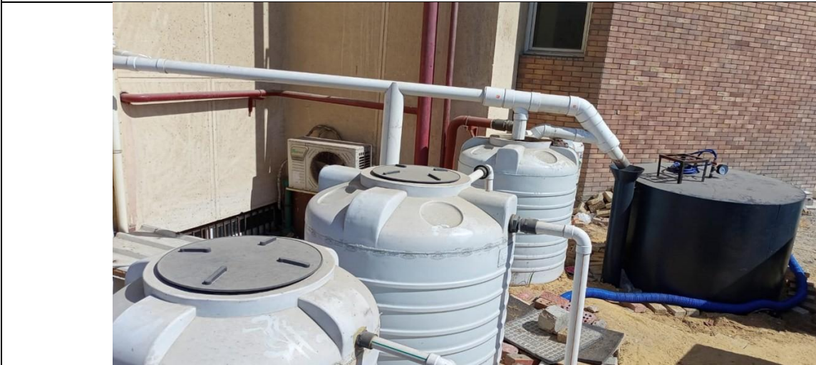
Wastewater treatment unit at the Faculty of Engineering
