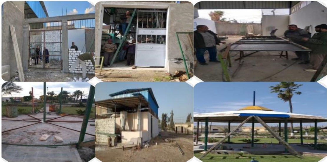
Recycling Program for both materials and equipment with metals and derivatives (Alexandria University, Egypt)
