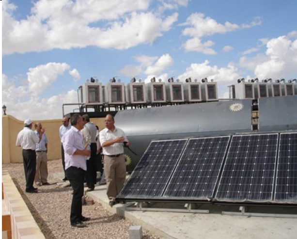
Innovative Renewable Energy RE-Multi-stage flash system (MSF) with salt precipitator and nanofiltration (NF-MSF) to pre-treat feedwater (RE-NF-MSF). Faculty of Agriculture, Alexandria University
