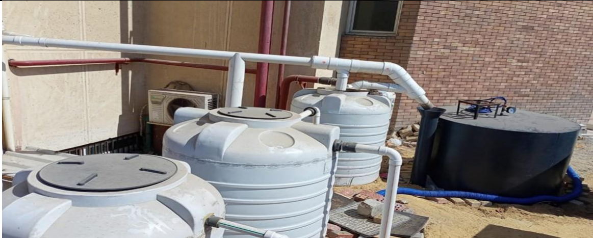
Wastewater treatment unit at Faculty of Engineering
