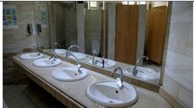
Supplying water taps with water conservation units (Alexandria University, Egypt)
