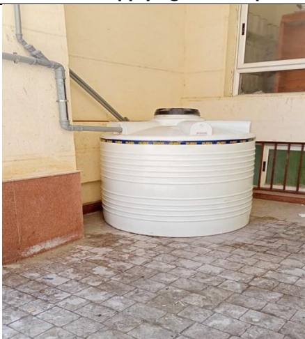
Supplying water taps with water conservation units (Alexandria University, Egypt)
