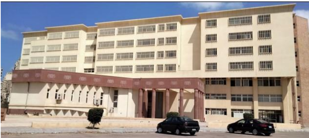
Green building implementation through the use of sun breakers in the SSP building at the Faculty of Engineering
