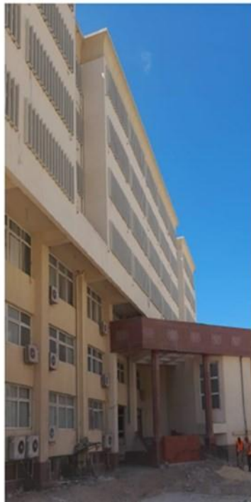
Photos of Faculty of Engineering SSP Building
