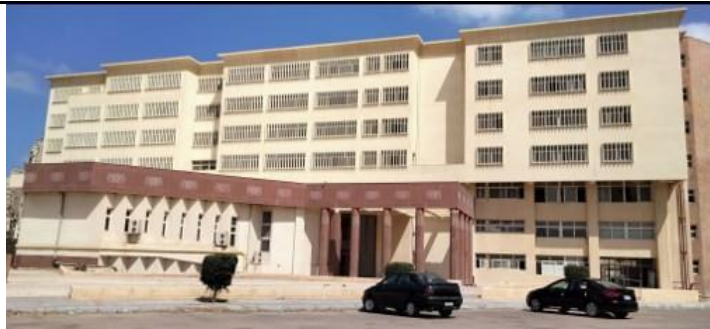
Green building implementation through the use of sun breakers in the SSP building at the Faculty of Engineering
