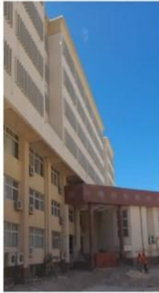
Photo of Faculty of Engineering SSP Building
