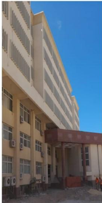
Photos of Faculty of Engineering SSP Building
