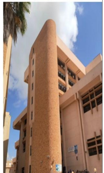
Photos of Faculty of Education Building
