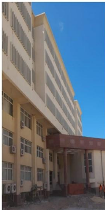
Photos of Faculty of Engineering SSP Building
