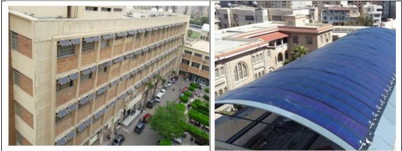
BIPV Façade Brise-Soleil System Solar Energy Project at the Faculty of Science (Alexandria University)
