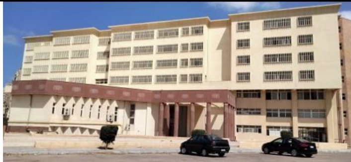
Green building implementation through the use of sun breakers in the SSP building at the Faculty of Engineering
