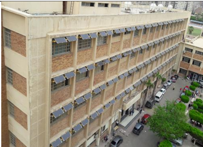
BIPV Façade Brise-Soleil System Solar Energy Project at the Faculty of Science (Alexandria University)
