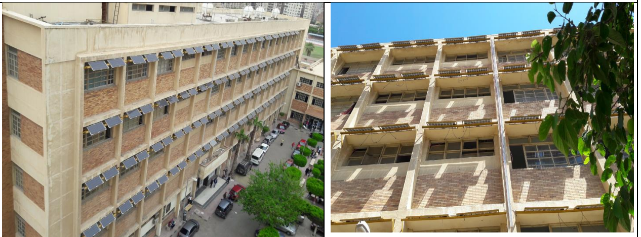
BIPV Façade Brise-Soleil System Solar Energy Center at the Faculty of Science (Alexandria University)
