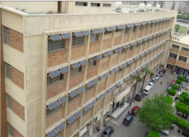
BIPV Façade Brise-Soleil System Solar Energy Project at the Faculty of Science (Alexandria University)
